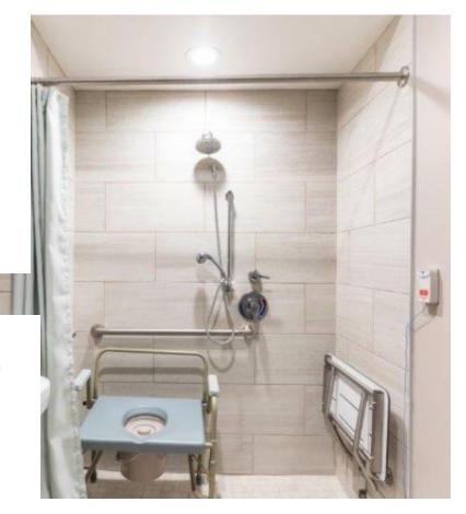
SPS 382.50(3)(b)5. Water provided to patient showers, therapeutic equipment and all types of baths shall be installed with pressure balanced and thermostatically controlled control valves...
